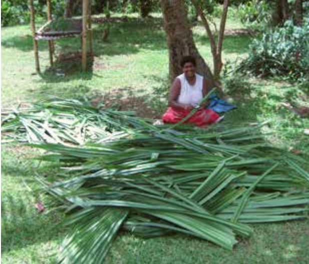
Preparing a roof, Fiji. Traditional building materials come from the land. Photo: Broeckmann/Misereor
