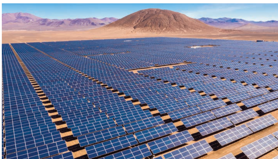
Solar energy PV power plant in Atacama, Chile. © Abriendomundo / Shutterstock
